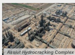
Assiut Hydrocracking Complex
